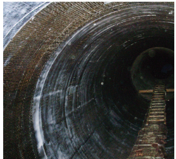
Tyfo® retrofit on water pipe
