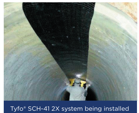
Tyfo® SCH-41 2X system being installed
