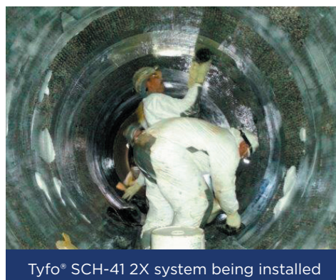
Tyfo® SCH-41 2X system being installed
