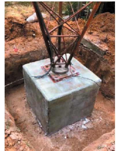
General view of foundation
