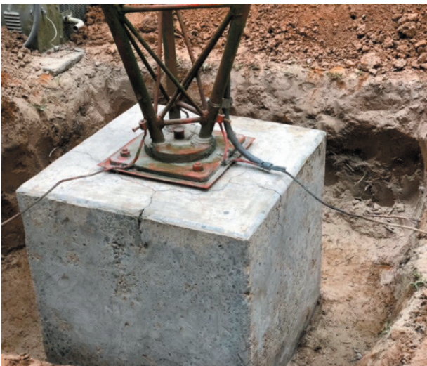
Concrete cleaned and prepped.
