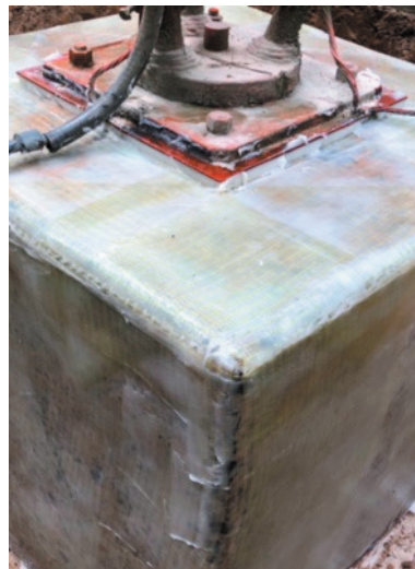
Concrete foundation with FRP applied
