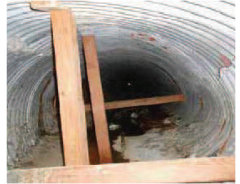
High-risk areas braced with timber.
