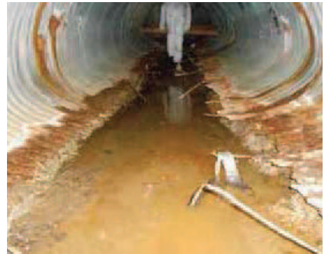
The repair began with excavating and cleaning.
