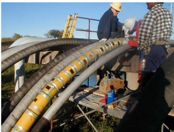
Clock Spring units being installed using the hand spool technique
