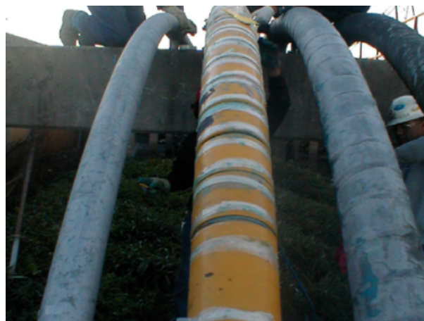
Coils cut to width to suit the bend radius
