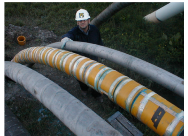
One of the completed bend repairs on one side of the canal crossing
