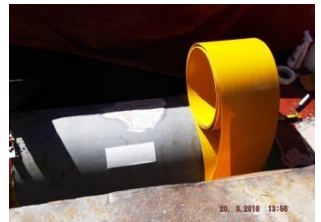
The Clock Spring composite sleeves are installed using the hand spool method.
