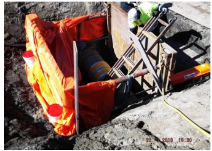
Clock Spring Repairs Crude Oil Pipeline
