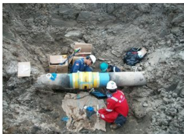
The team completes the repair with the installation of the third coil.
