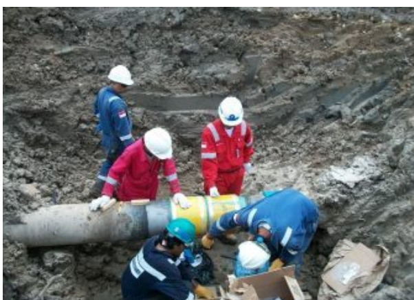
Certified installers place bridge units on each side of the weld.
