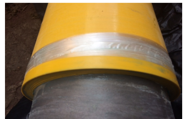
Edge of completed repair.
