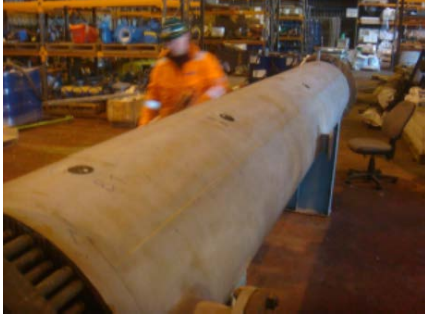
Sensors were permanently installed with high temperature adhesive.
