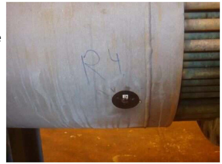
Sensors were positioned seven inches inside the boundaries of the repair.
