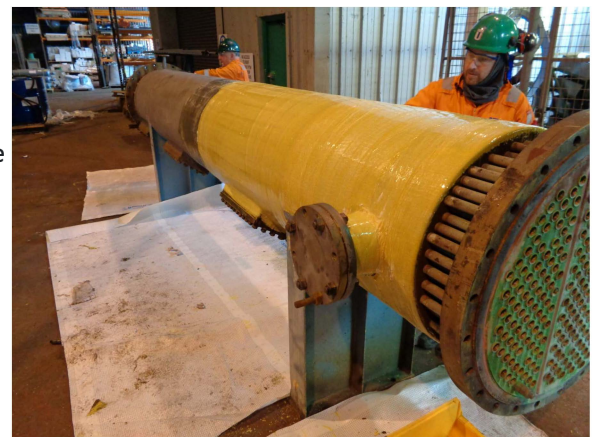
With the WAND system, thickness measurement data can be accessed wirelessly through the ThermoWrap® MT repair.
