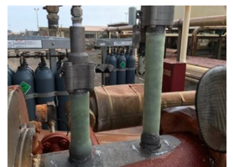
Pin Hole Completed repair
