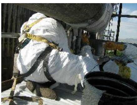
Converting nozzle area with composite box
