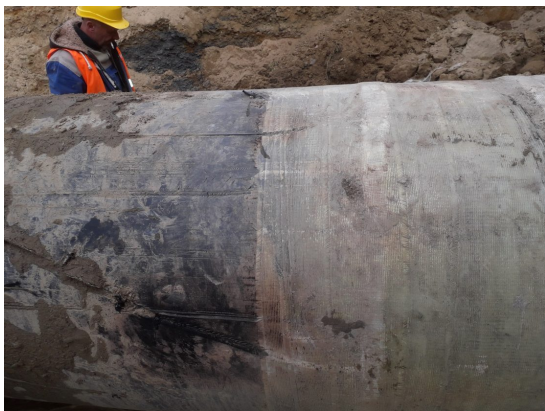
The two-layer Contour system, installed along a 700 mm (27.6 inch) section of pipeline, acts as mechanical protection over welded joints.
