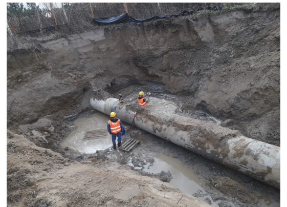
Clock Spring trained and certified installers assess the 1,000-mm (39.3-inch) carbon steel natural gas line.
