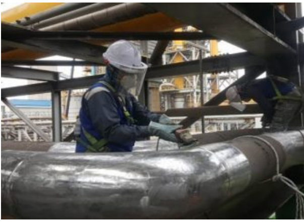
Installers from Dong-buk E&C prepare the surface of the pipe for the Contour repair.
