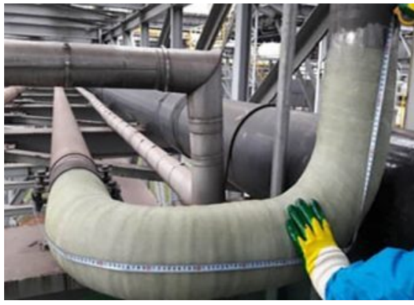
The installation team applies the Contour fiberglass cloth to the pipeline.
