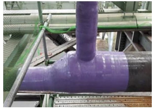
The Clock Spring Contour repair restores the line to safety.
