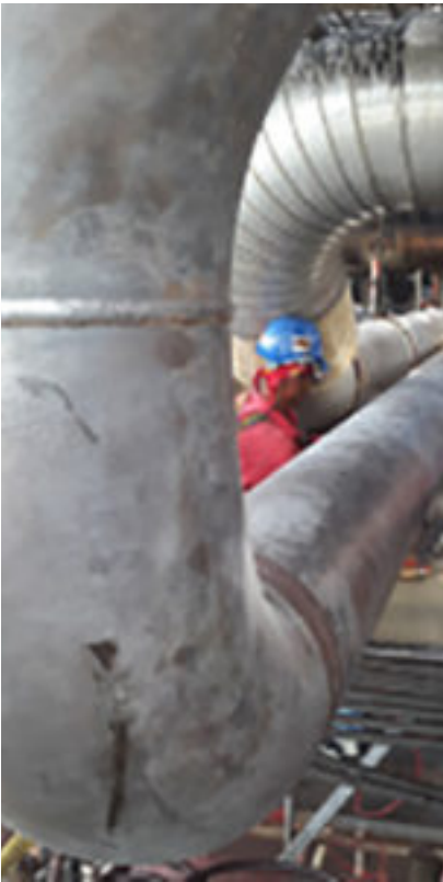
DiamondWrap Internal Corrosion Repair
