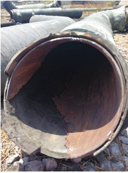
Repair Forms Long Lasting New Pipe
