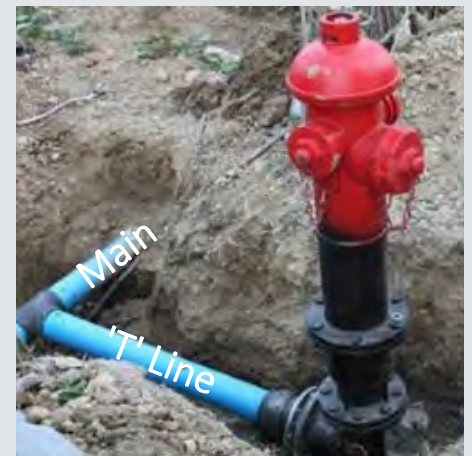
Typical fire hydrant set up
