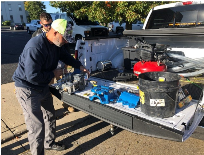
AVT's Tom Heylin preparing the EZ Valve for fitting
