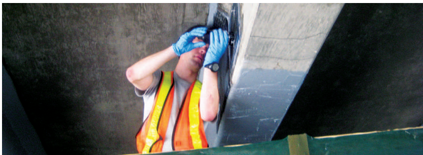
On-site adhesion testing ensuring quality assurance of the Tyfo® SCH system and the Fibrwrap installer's workmanship
