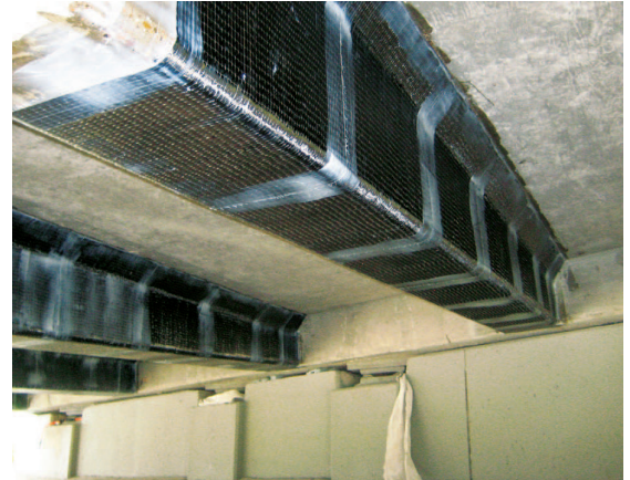
Installed Tyfo® SCH system at critical shear zones
