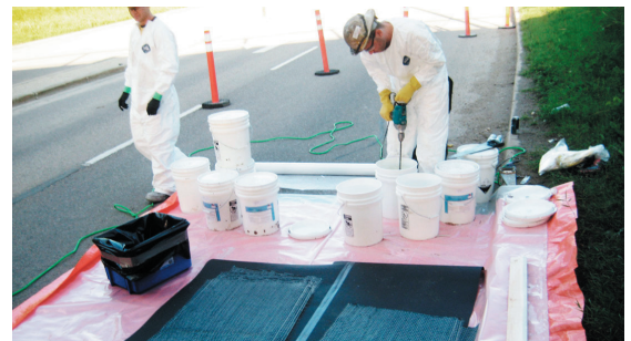
Fibrwrap® certified installers mixing and safely preparing the TYFO® SCH system with minimal site impact
