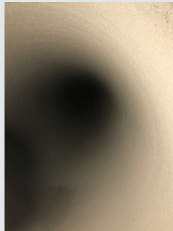
During: Completed installation of GeoSpray HCE gave the sewer a new liner which will last for decades
