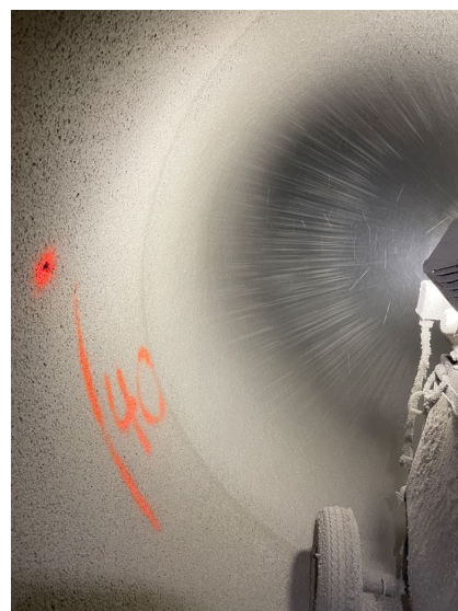
GeoSpray HCE installation via centrifugal force
