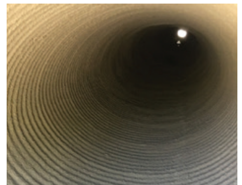
Completed repair over a formerly separated joint.
