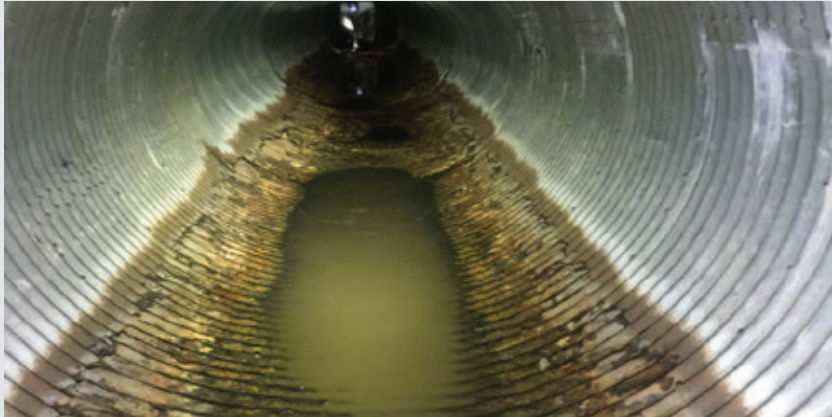
Corroded invert.
