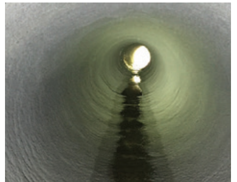
Completed rehabilitation using GeoSpray mortar.
