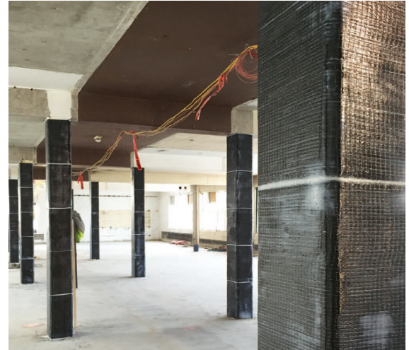
Columns with Tyfo® SCH-41 strengthening system
