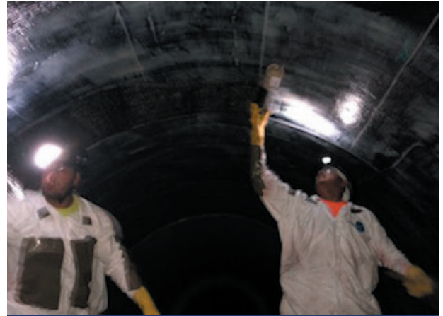
Tyfo(r) CFRP being placed in the hoop direction.
