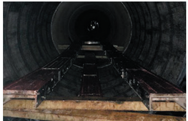
Scaffolding is used to provide work access to apply the Tyfo® CFRP product
