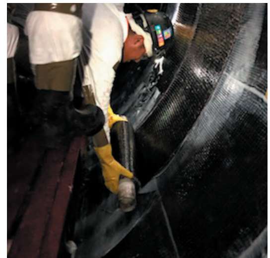
Tyfo® unidirectional carbon fiber being placed and oriented in the hoop direction on the 120-inch PCCP pipeline
