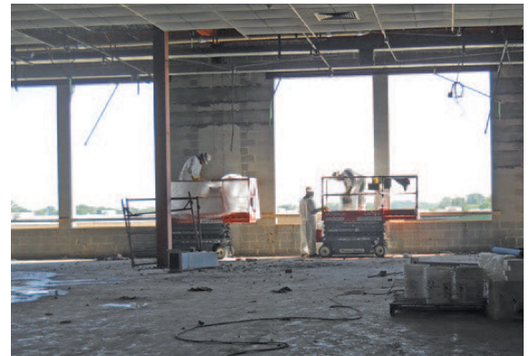
CMU Walls with Tyfo® SEH-51A System
