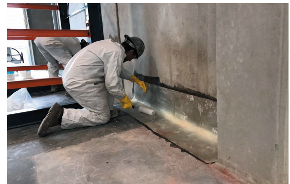
FRP installation at joint
