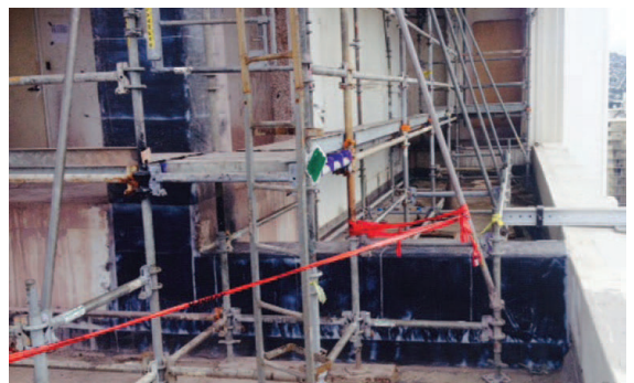
Tyfo® system application
