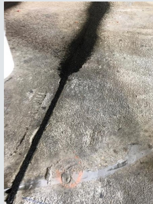
8. Aggregate was broadcast onto wet gel, and then excess was removed after cure of sealant. This step was an option selected to enhance adhesion of traffic coating to follow.
