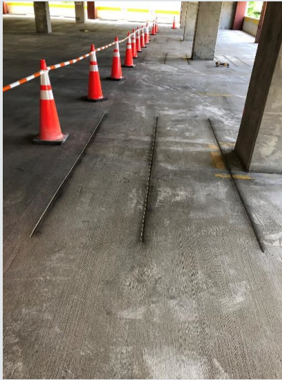
1. Saw cuts were made along columns in preparation for the NSM CFRP bars.
