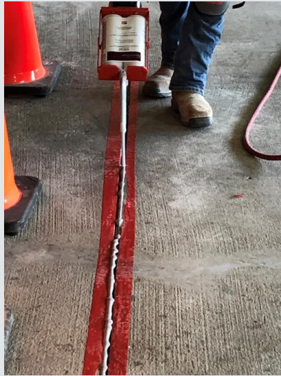
7. RenewWrap NSM Gel applied over inserted rod and tooled flush with substrate.
