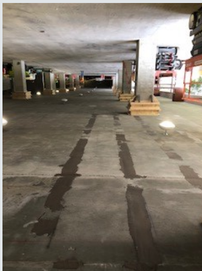
4. The slab preparation is completed prior to the application of the RenewWrap CFRP system.
