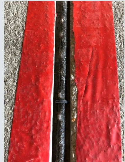
4. O rings applied to 3/8" NSM CFRP bars to provide proper placement into the cut.
