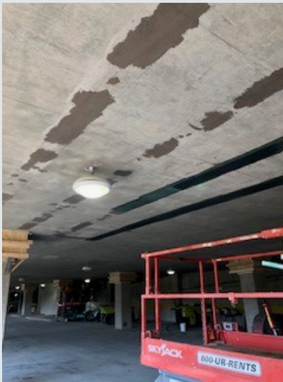
1. Strengthening of parking deck partially completed.
