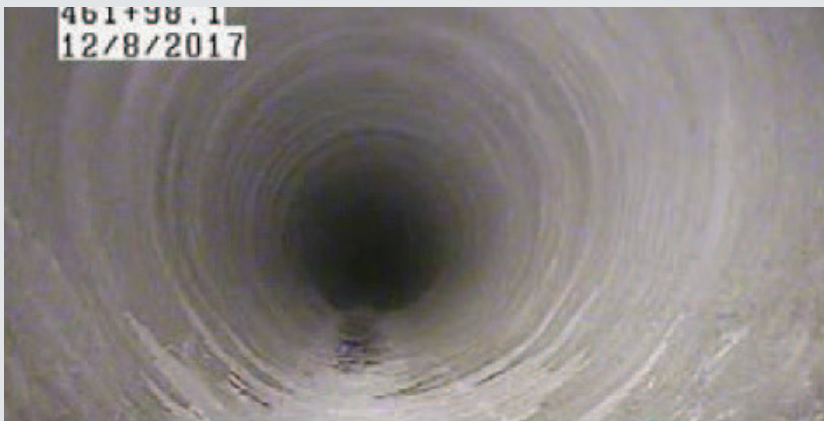
CCTV footage of completed rehabilitation.
