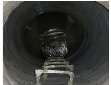
Rehabilitated vertical manhole structure.
