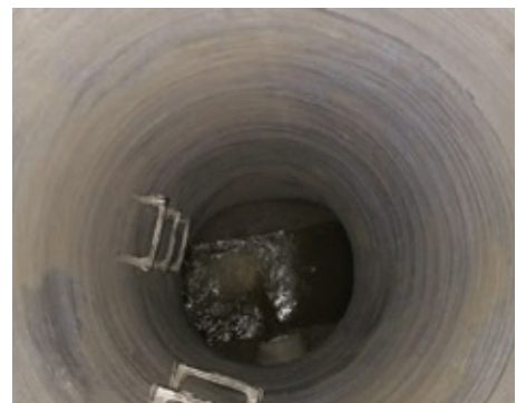
Completed manhole rehabilitation.
