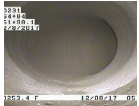
CCTV footage of curved section of pipe repaired.
