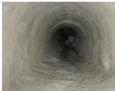
Arched brick pipe after completion.
