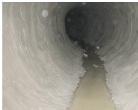
Circular brick pipe with curvature after completion.
