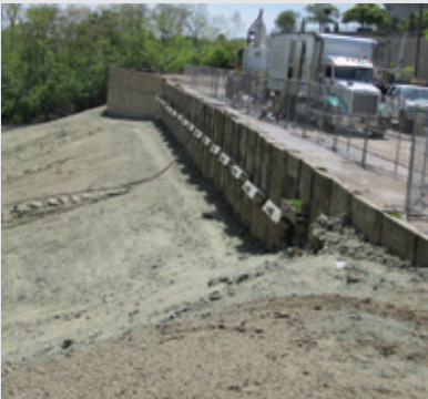
Extended working distance from material platform to repair site.
