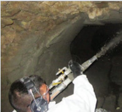
GeoSpray geopolymers being applied by hand spray to lock in existing brick and stone.
