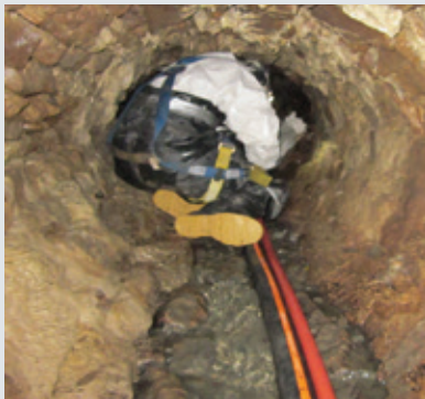
Hand-repairing of infiltration.
