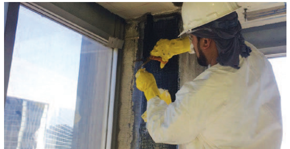
Tyfo® system application
