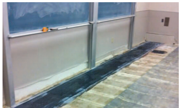
Tyfo® system application
