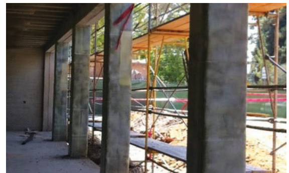
Tyfo® SEH-51A system applied to columns
