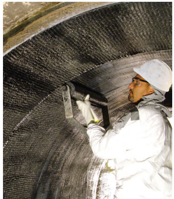
CFRP application to interior pipe
