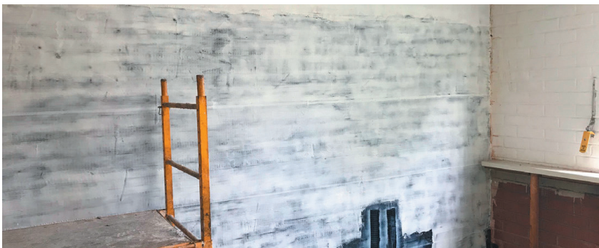
Finalizing the FC/C fire protection system
