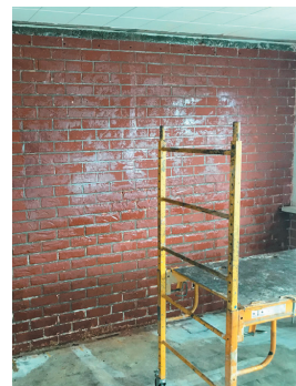
Wall to be retrofitted - before shot
