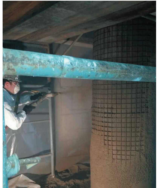
Shotcrete being applied to the column
