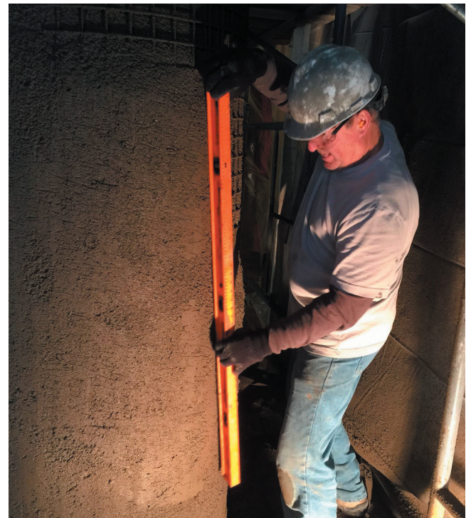
Finishing the shotcrete
