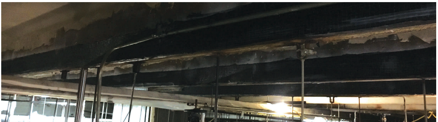
Double tee strengthening at line 1/2
