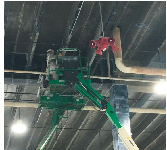
Double tee, girder and column strengthening at retort line
