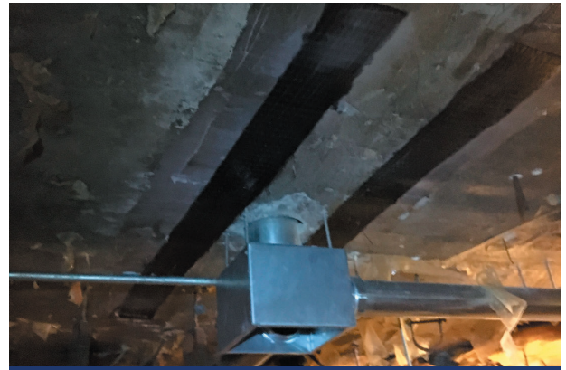
Underside of the slab positive flexural strengthening
