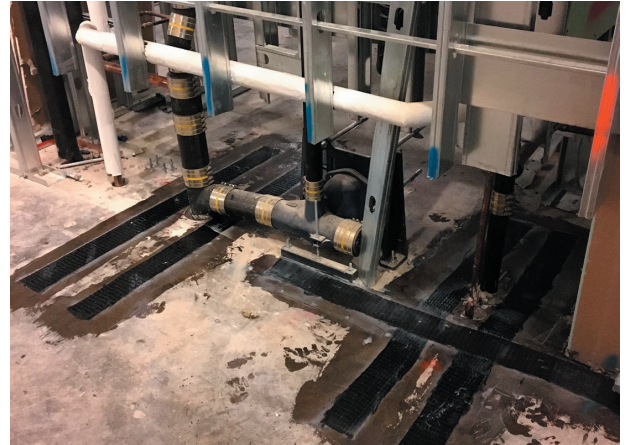
Strengthening in both transverse and longitudinal directions
