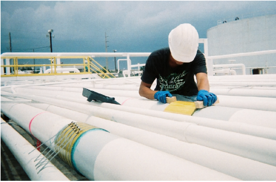
Technician aligns Snap Wrap coils prior to tightening
