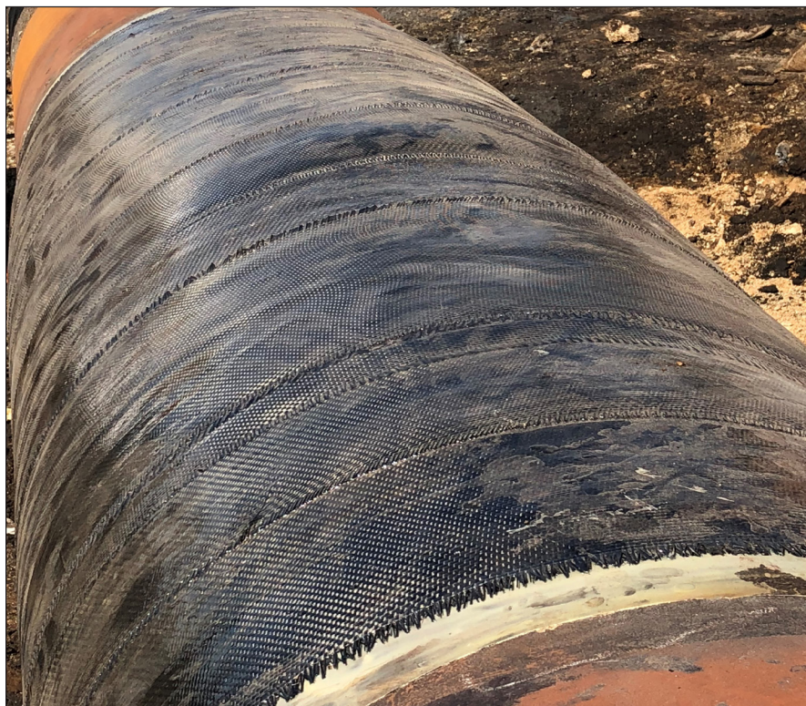
A line damaged in an explosion is wrapped with 26 layers of DiamondWrap and restored to safe service.
