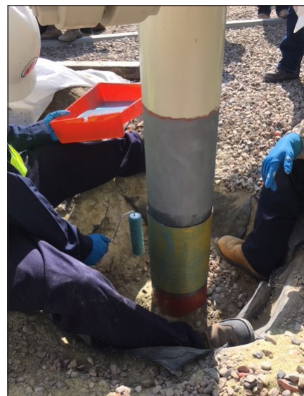
Installers secure Snap Wrap to strengthen a pipe and protect it at the air/soil interface.
