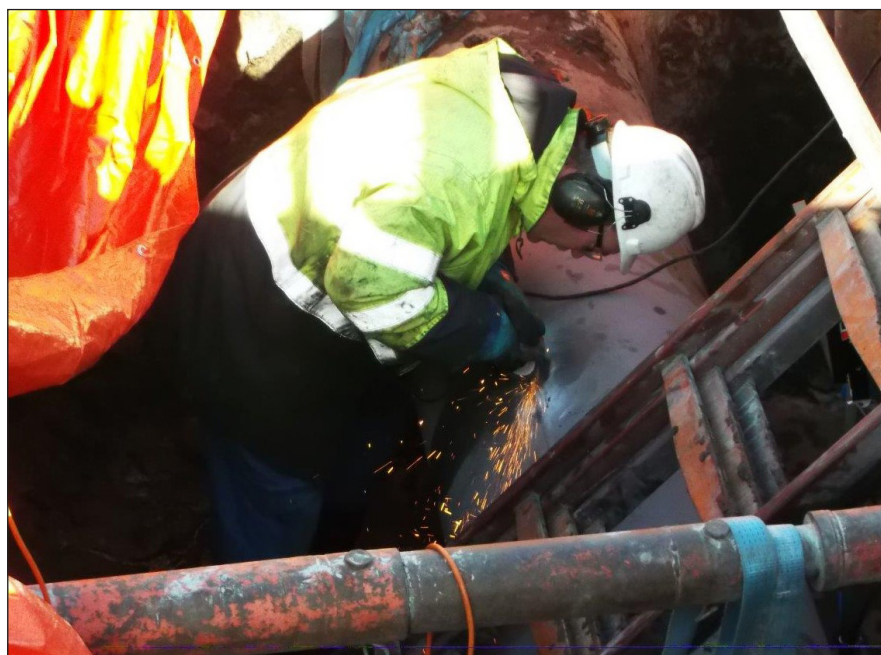
Technicians remove the crack in the seam weld with a grinder to prepare the surface of a carbon steel crude oil pipeline for a composite repair. Photos courtesy of CSNRI
