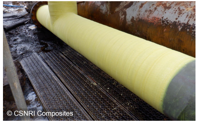
Figure 3. CSNRI's ThermoWrap MT restores through-wall defect.
