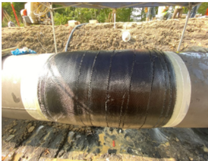
Figure 7. Reinforcement of a girth weld with the Atlas UA carbon fibre repair system in a region with active geohazard threats.
