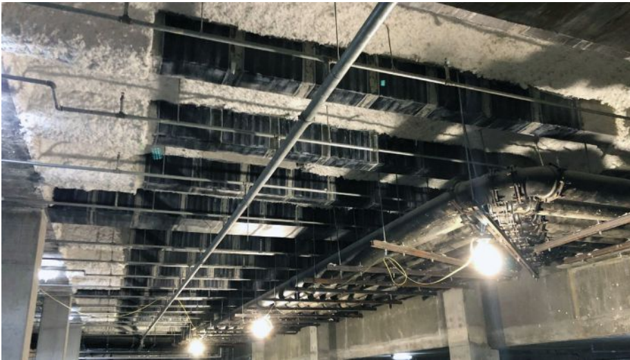
To supplement the shear capacity of the museum's existing reinforced concrete floor beams, the project team oriented a unidirectional carbon fiber system in a "U-Wrap," with the primary fibers running transversely to the axes of the beams.
