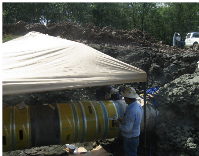
Figure 1. Workers installing Clock Spring's Pipe Support.
