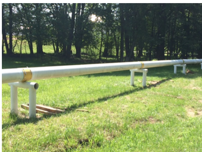
Figure 3. Clock Spring's Pipe Support applied to refined product pipe.
