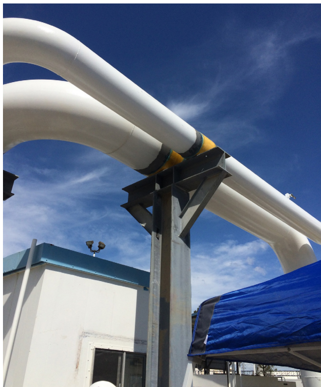
Figure 2. Clock Spring's Pipe Support applied to a liquid pipeline.
