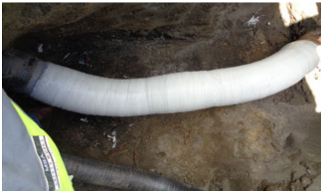
Figure 2. Pipeline repaired with the A+ Wrap™ repair system.
