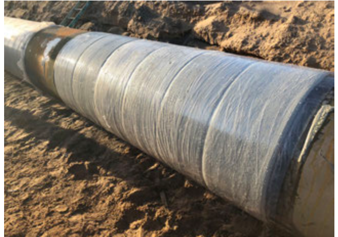
Figure 3. A+ Wrap system repair utilising the offset method.
