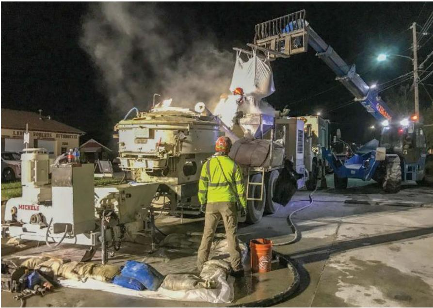
and 3 in. in a 130-lf section of steel plated tunnel. In addition, the crew applied 1 in. in 50 vf manhole shaft, covering a total of 11,250 sq ft, and approximately 325 lf of geopolymer fill in the belly of the pipe. In total, 670,000 lbs of geopolymer mortar was applied on the project.
