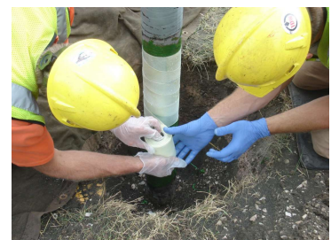
SynthoGlass® applied over epoxy coating reduces time invested in coating inspection.
