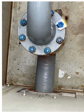
SynthoGlass® used to protect vault wall link seal.
