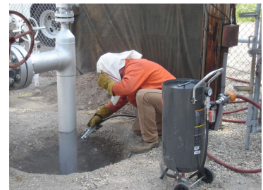
Abrasive blasting used to prepare for application of epoxy and SynthoGlass®.
