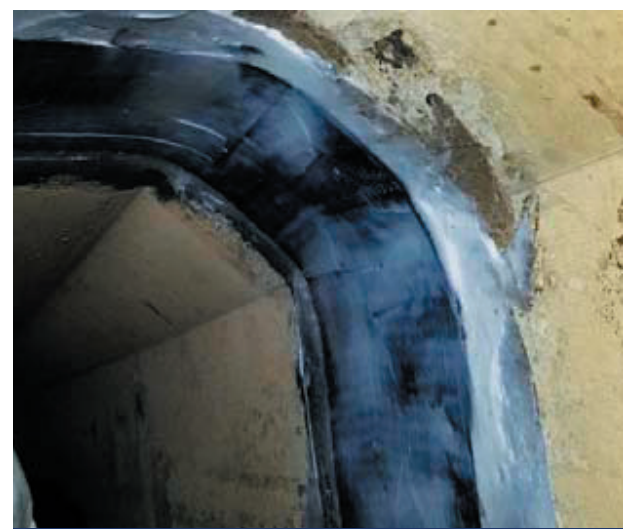
CFRP joint repair
