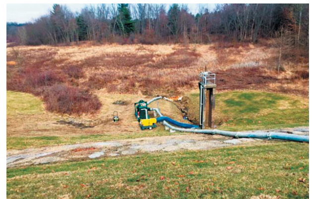
Bypass pumping setup
