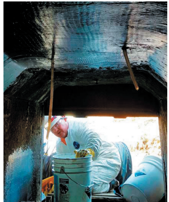
CFRP concrete repair
