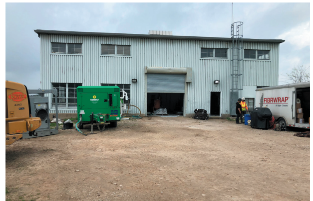
Lake Houston pump station - Boyer
