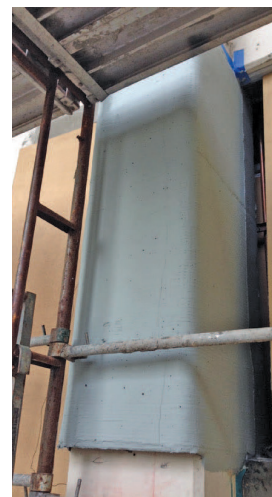
Column with Tyfo® SCH-41 system applied
