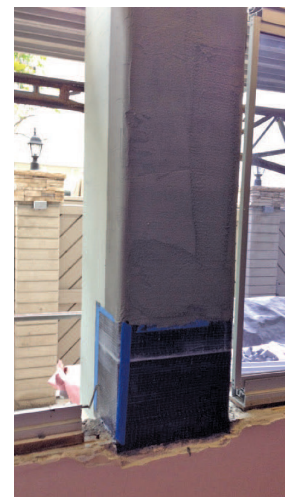
Column with Tyfo® SCH-41 system applied
