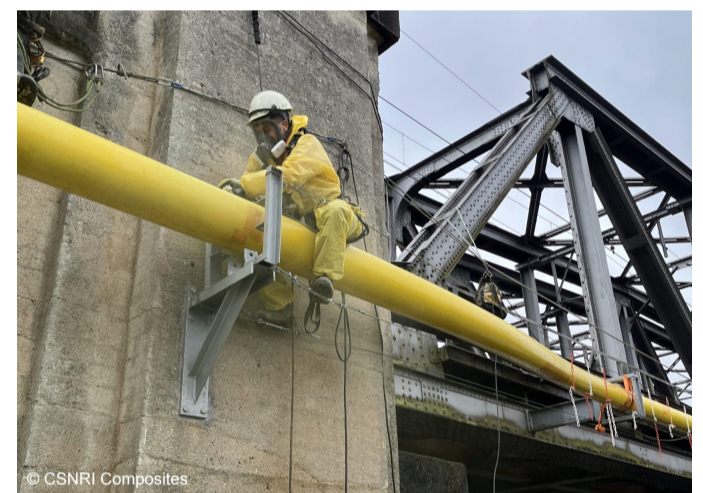
Before Pipe Support Installation
