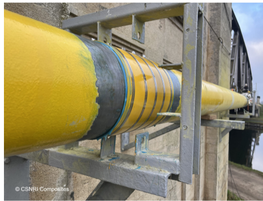
The Pipe Support system creates a non-corrosive environment where the pipe comes into contact with the support, repairing defects and providing protection against future damage.
