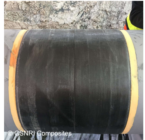
The completed Atlas repair fully restored structural integrity and pipe function.
