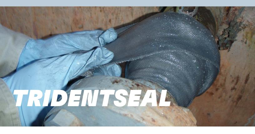
Designed to address the need for simple, instant, tamper-proof, live leak repair on gas piping, TridentSeal permanently seals active gas leaks ≤125 psi (8.6 bar) without interruption to service.
